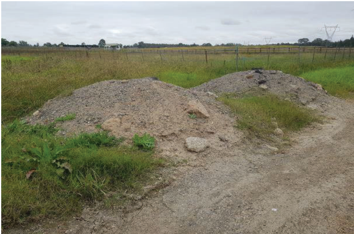
Image 6.10.5 View of stockpiles (SP2 and SP3) containing silt and aggregate with demolition waste inclusions
