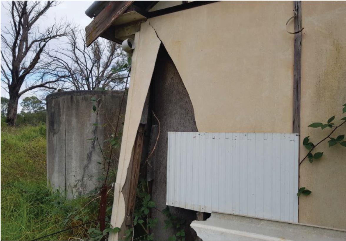
Image 6.9.1 View of broken walls of old fibro cottage
