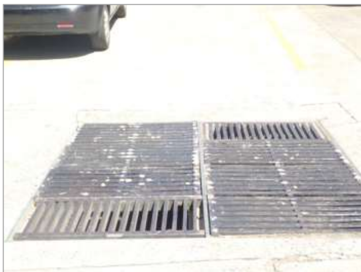
Figure 19. One of the access covers to the stormwater channel containing the former creek.
